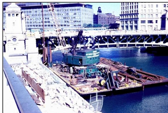
Figure 6-3 Above Water Equipment on Barge
