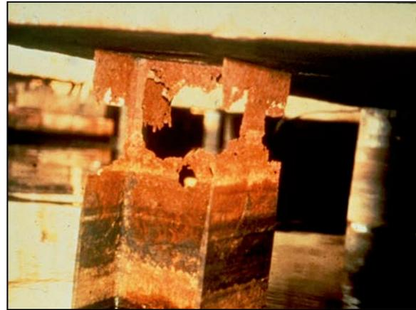
Figure 3-1 Steel Deterioration Resulting from Corrosion
