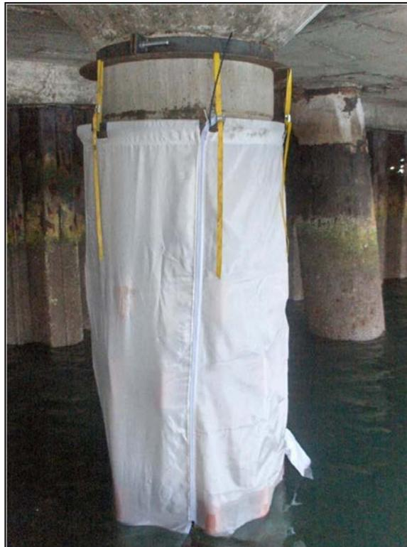
Figure 8-16 Fabric Form Installation
