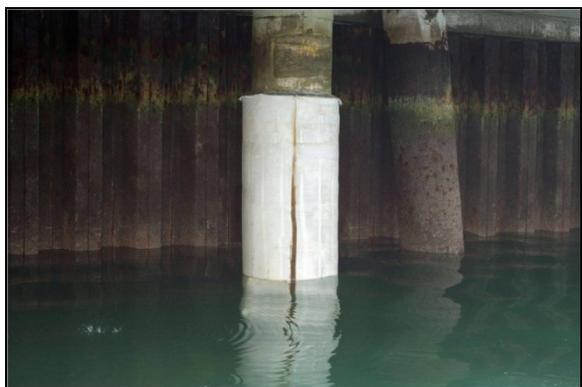
Figure 8-19 Completed Fabric Form Jacket
