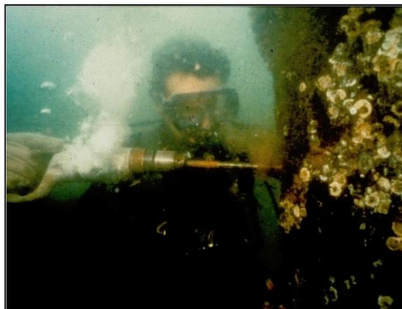
Figure 6-7 Pneumatic Drill
