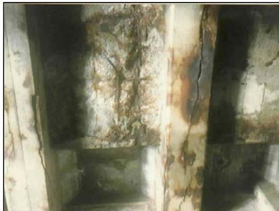
Figure 3-6 Cracks Along Reinforcing Bars
