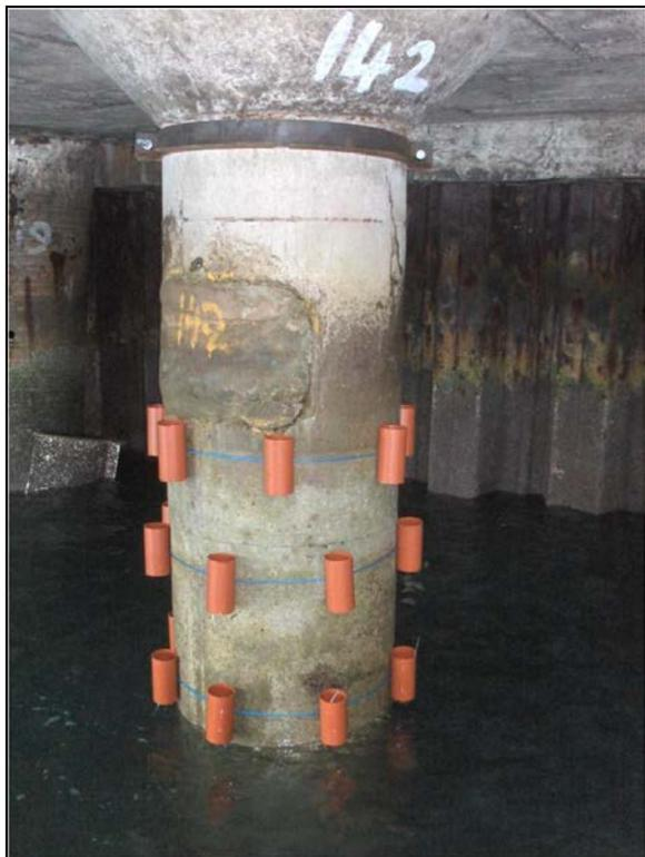
Figure 8-15 Formwork Spacers in Place
