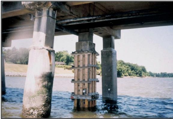
Figure 8-22 Completed Composite Jacket (Back Pile) and Jacket Read to be Pumped (Middle Pile). The Stiffening System is in Place on the Middle Pile Due to the Flexibility of the Fiberglass Jacket Form.
