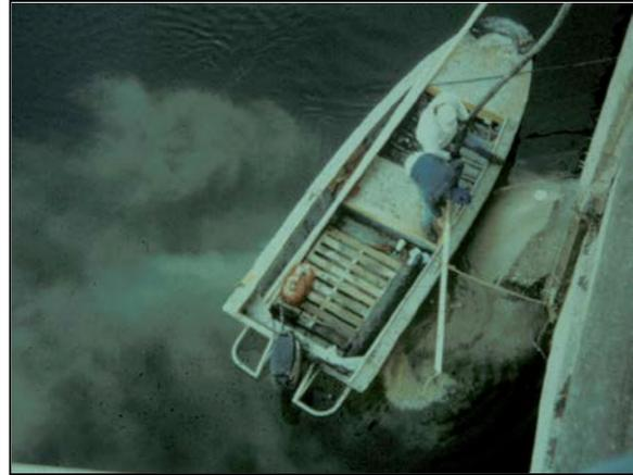
Figure 5-4 Grout Discharge into River
