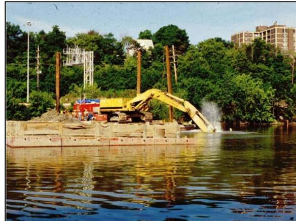
Figure 6-14 Hydraulic Excavator Performing Underwater Excavation
