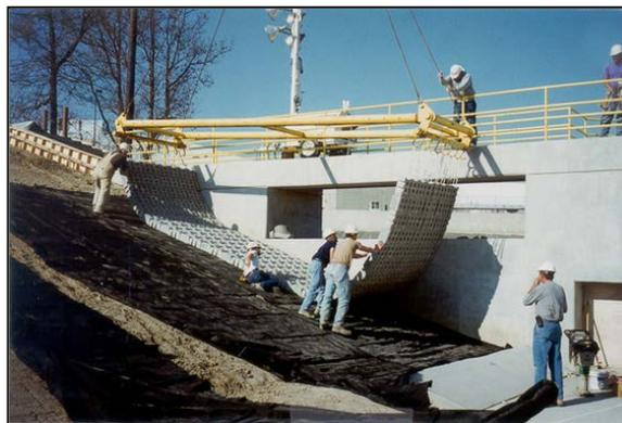
Figure 7-15 Articulated Concrete Block System Being Installed
