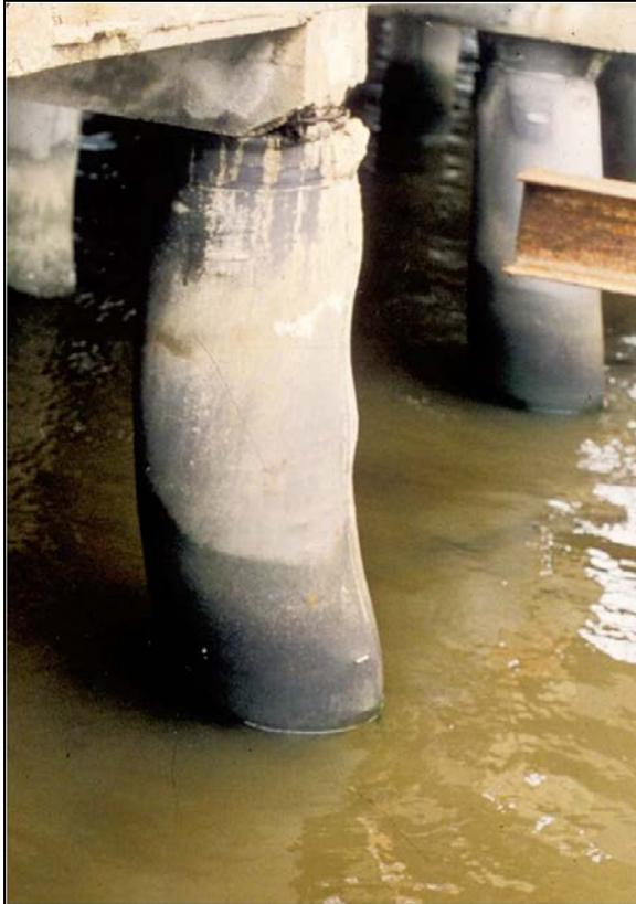
Figure 8-25 Displaced Fabric Formed Pile Jacket Due to Lack of Spacers and Uneven Grout Placement
