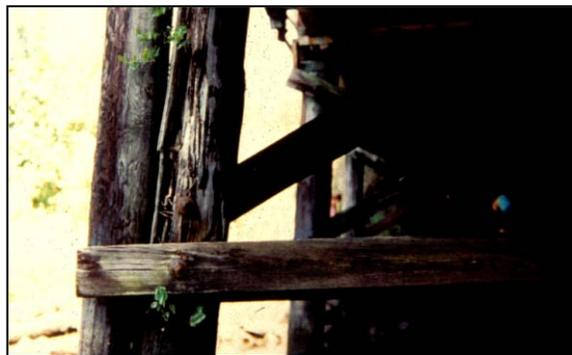
Figure 8-2 New Pile Driven Outside of Damaged Pile
