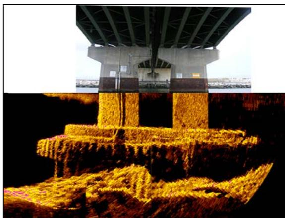
Figure 3-4 Undermining of Footings
