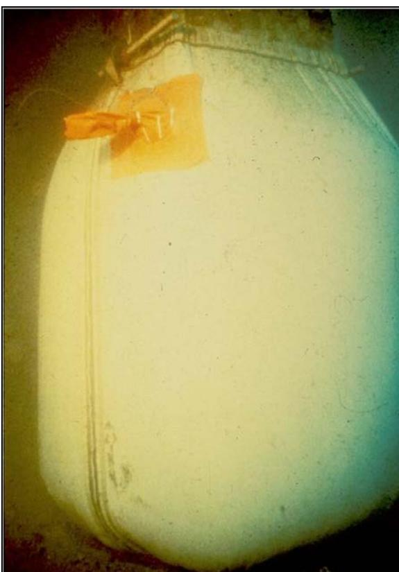
Figure 8-20 Completed Underwater Fabric Form Repair
