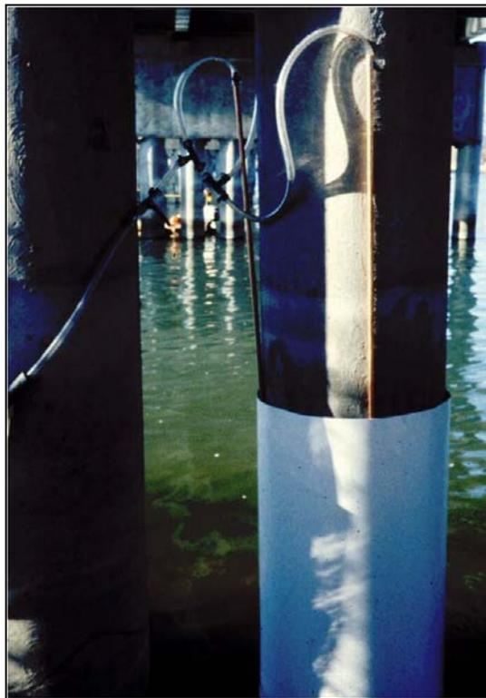
Figure 8-24 Epoxy Placement Pipes in Form
