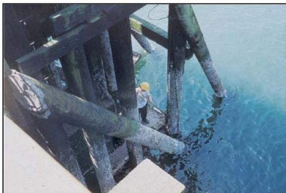
Figure 8-8 Pile Cleaning
