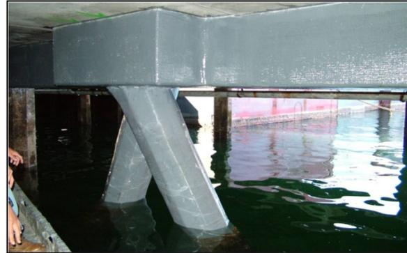
Figure 8-29 FRP Strengthening of Concrete Piles and Pile Cap
