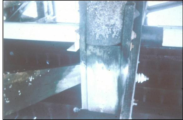
Figure 8-7 Pile Replacement Using Splice Plates
