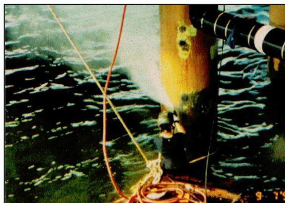
Figure 6-12 High Pressure Water Jet
