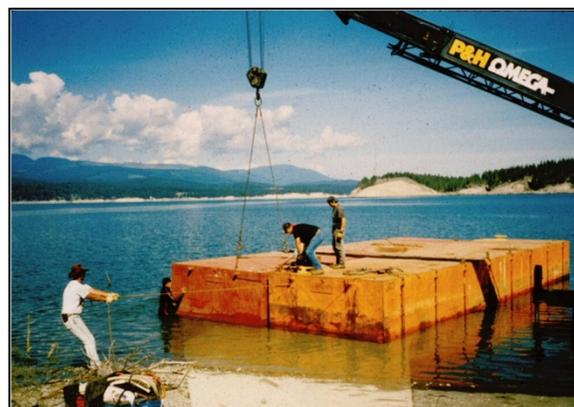
Figure 6-4 Sectional Barges Being Assembled
