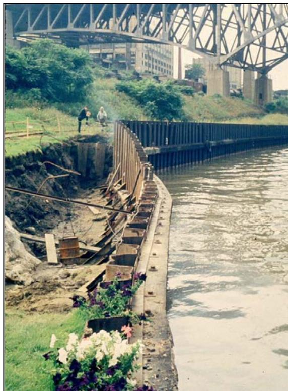
Figure 8-30 Sheet Pile Wall Failure
