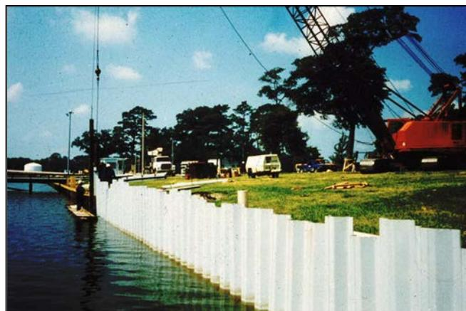
Figure 4-9 Polymer Sheet Pile Wall
