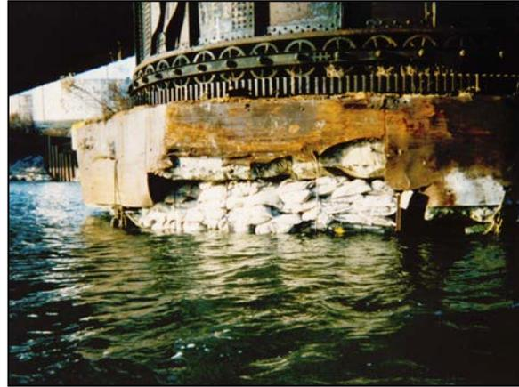
Figure 7-4 Bagged Concrete Emergency Repairs to Swing Pier
