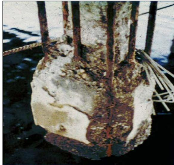
Figure 3-10 Concrete Pile During Repair
