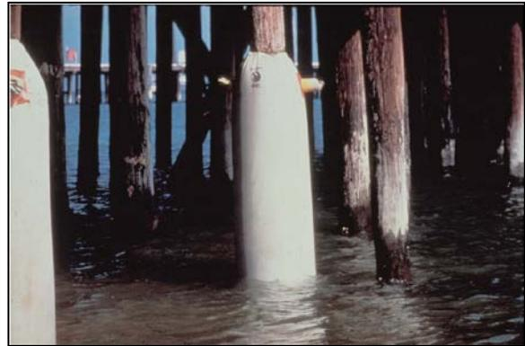
Figure 8-13 Typical Fabric Bag Concrete Pile Jacket on Timber Pile
