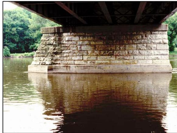
Figure 7-8 Concrete Encasement of Stone Pier
