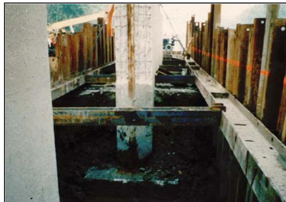
Figure 5-7 Cofferdam Used for Pier and Foundation Extension
