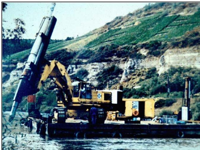
Figure 6-15 Specialized Underwater Hydraulic Hammer
