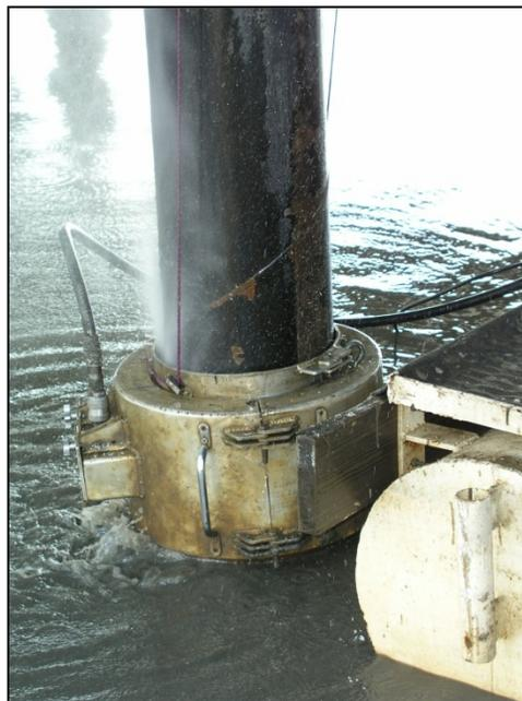
Figure 6-16 Contractor Built Pile Cleaning System
