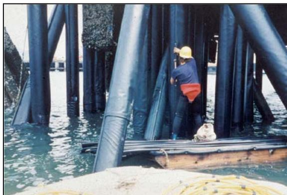
Figure 8-9 Pile Wrap Installation
