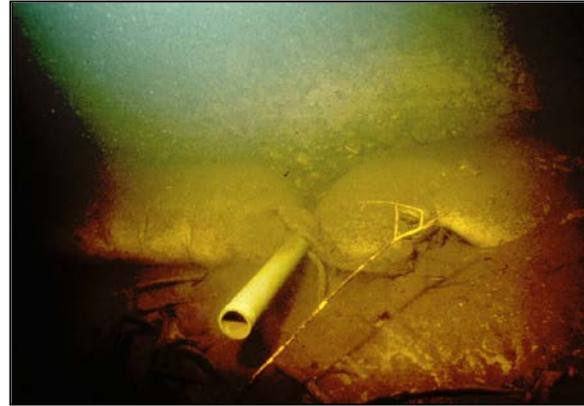
Figure 7-10 Grout Bag and Inlet Pipe
