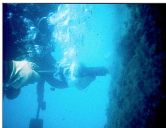
Figure 6-6 Pneumatic Needle Gun
