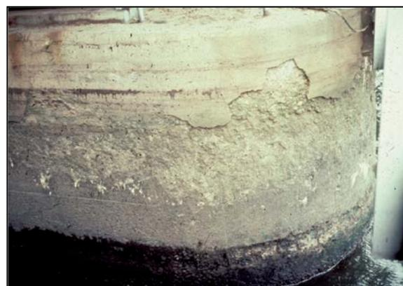
Figure 3-5 Deteriorated Concrete
