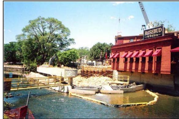
Figure 5-8 Bridge Pier with Dike Constructed of Soil, Traffic Barriers, and an Impervious Membrane
