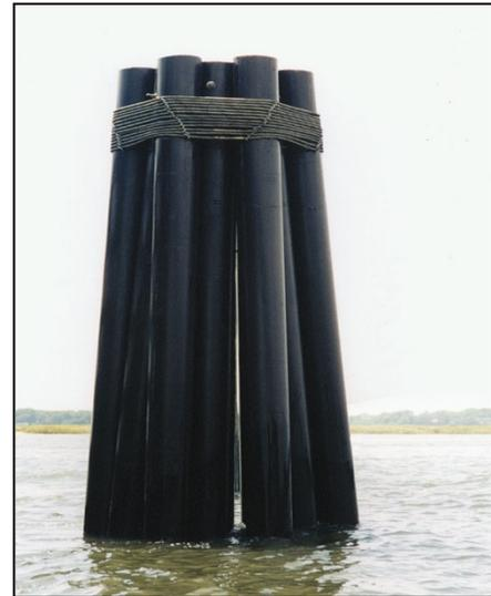
Figure 4-7 Polymer Pile
