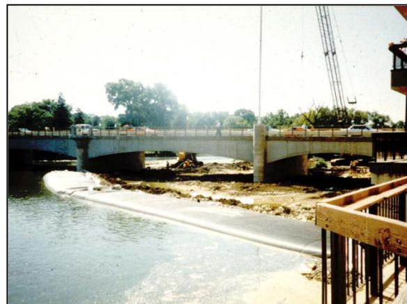
Figure 5-9 Water Filled Tubular Barrier
